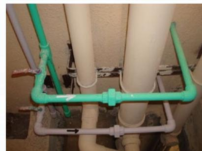
Pipe colour coding and arrow marking.
