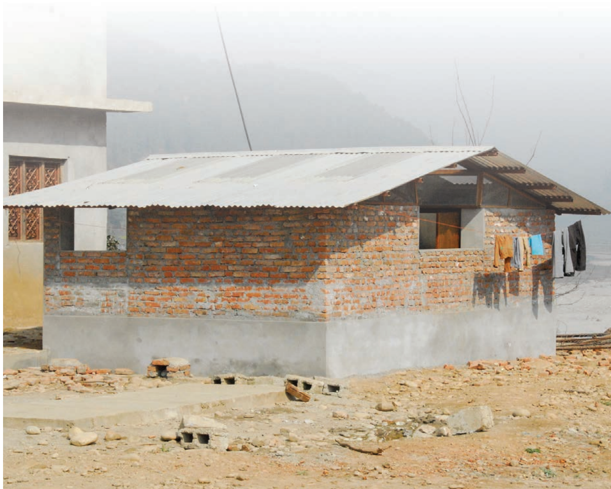
Stage 1 – Completed girls toilet block
