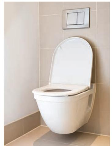
In the mid 1980, a 6 lpf low-flush closets began to be installed in India. The dual flush closets using 3 liters for half flush and 6 liters for full flush are voluntarily (and sometimes due to mandates) adapted widely. It is estimated that a closet is flushed full once, followed by two half flushes. That brings the water consumption to 4 lpf. Currently the 3-6 dual flush has approximately 60 to 70% market penetration.
