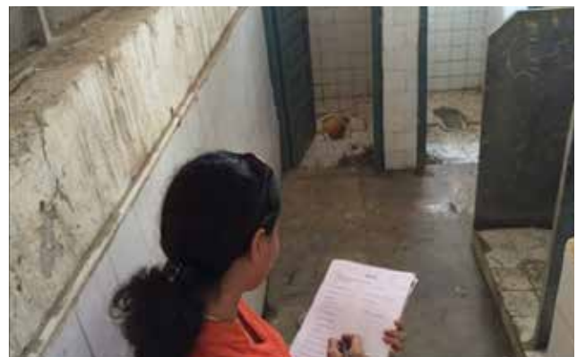
Swathi using the Feasibility checklist inside a school toilet area in Nashik
